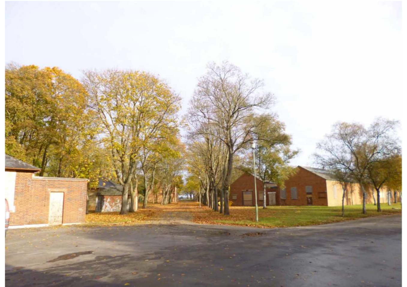
Fig 1: View towards Building 90 from the site entrance
