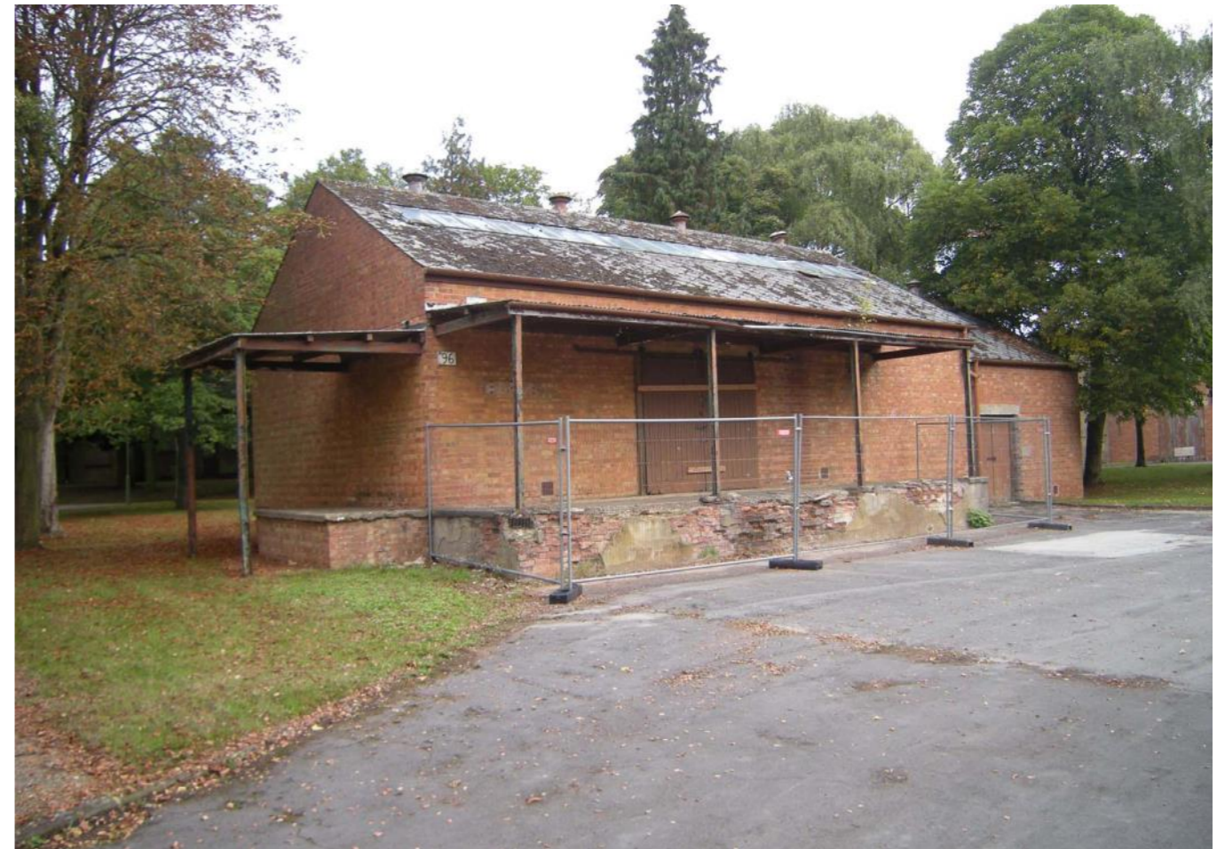
Fig 7: The Lubricant Store (Building 96)
