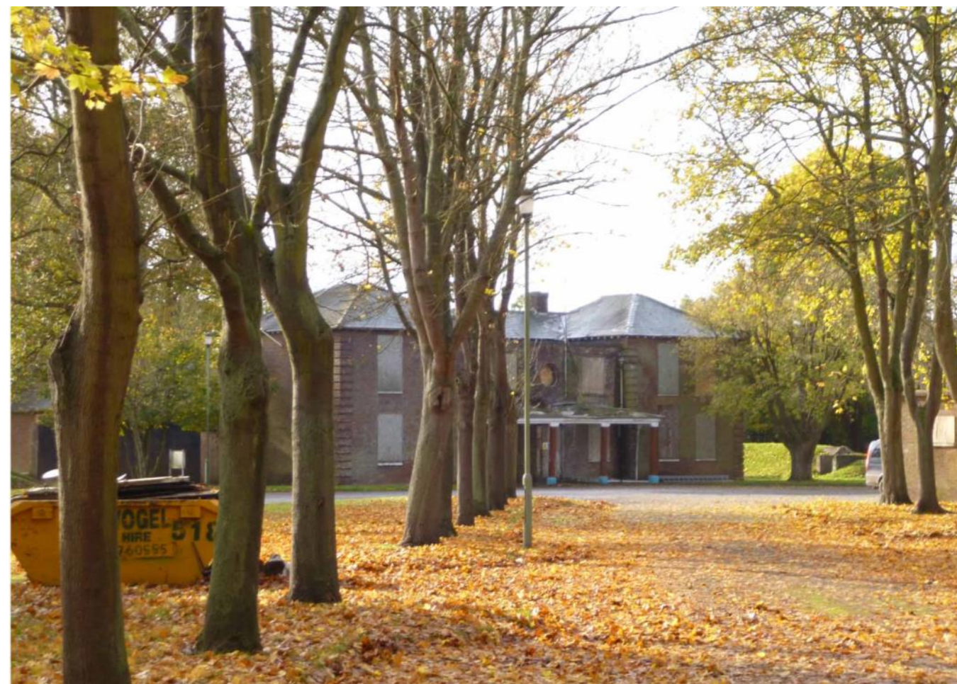
Fig 6: The Station Offices (Building 147)
