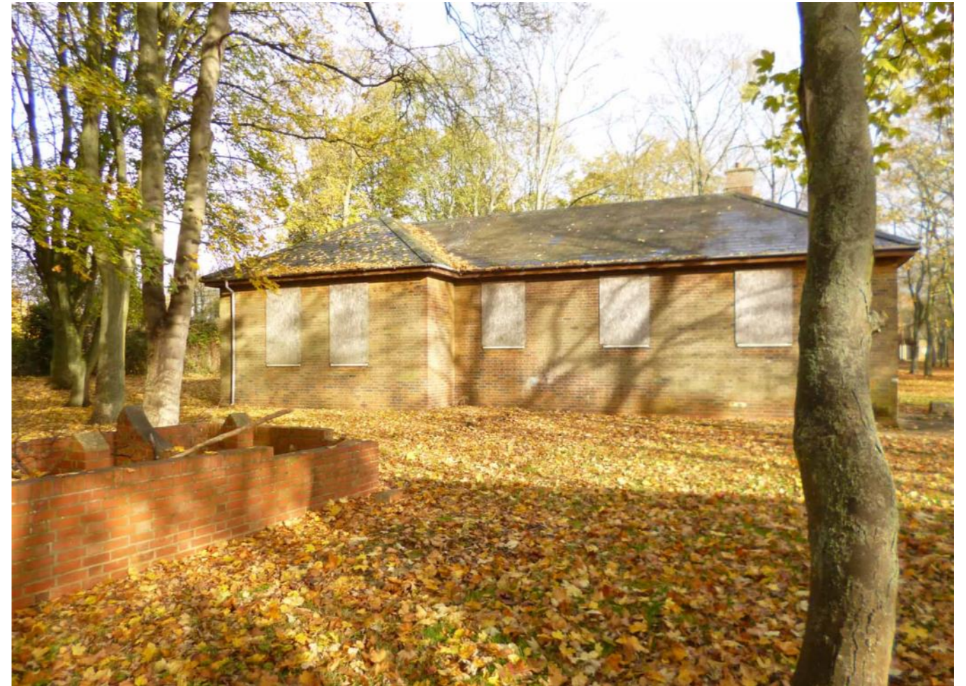
Fig 5: View of The Fire Party House (Building 87) from the South
