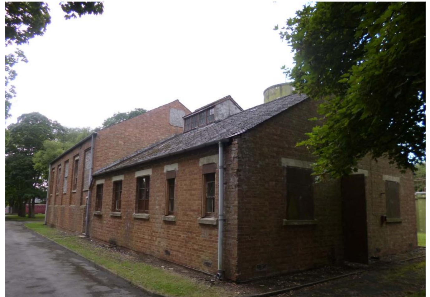
Fig 14: View from north of the site, Old Power House (Building 82)
